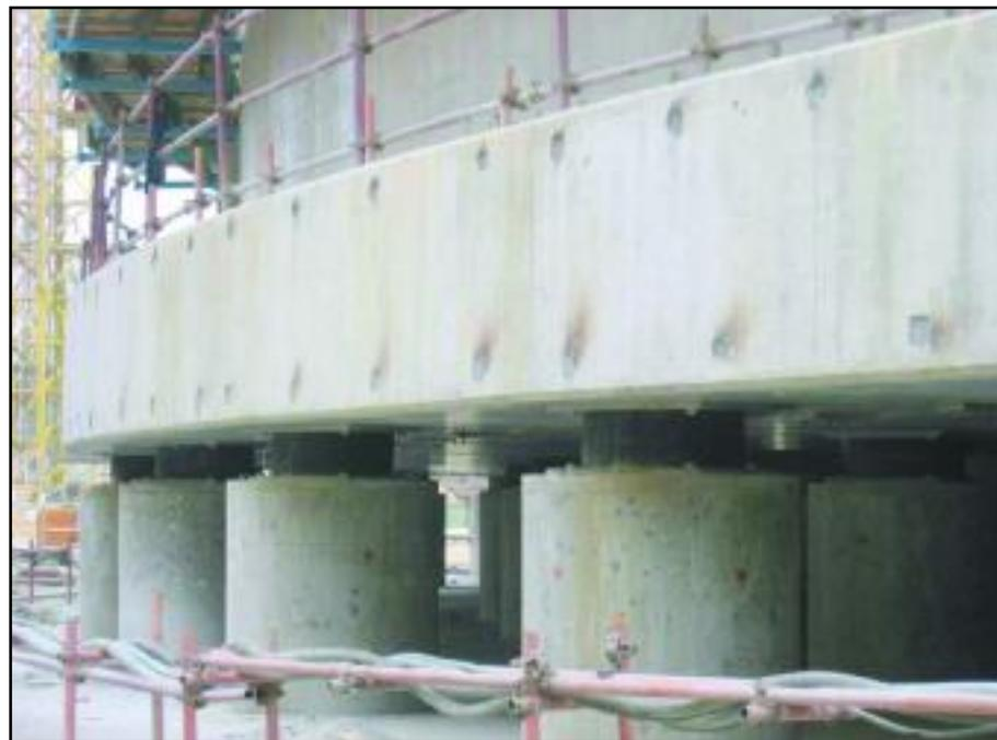
TARRC engineers were able to support, through Rubber Consultants, the successful bid of a Malaysian company for the supply of high damping rubber isolators for two liquefied natural gas tanks in China. The backing of the Consultancy was an essential prerequisite to the award of the contract, the largest such contract awarded to a Malaysian manufacturer.
